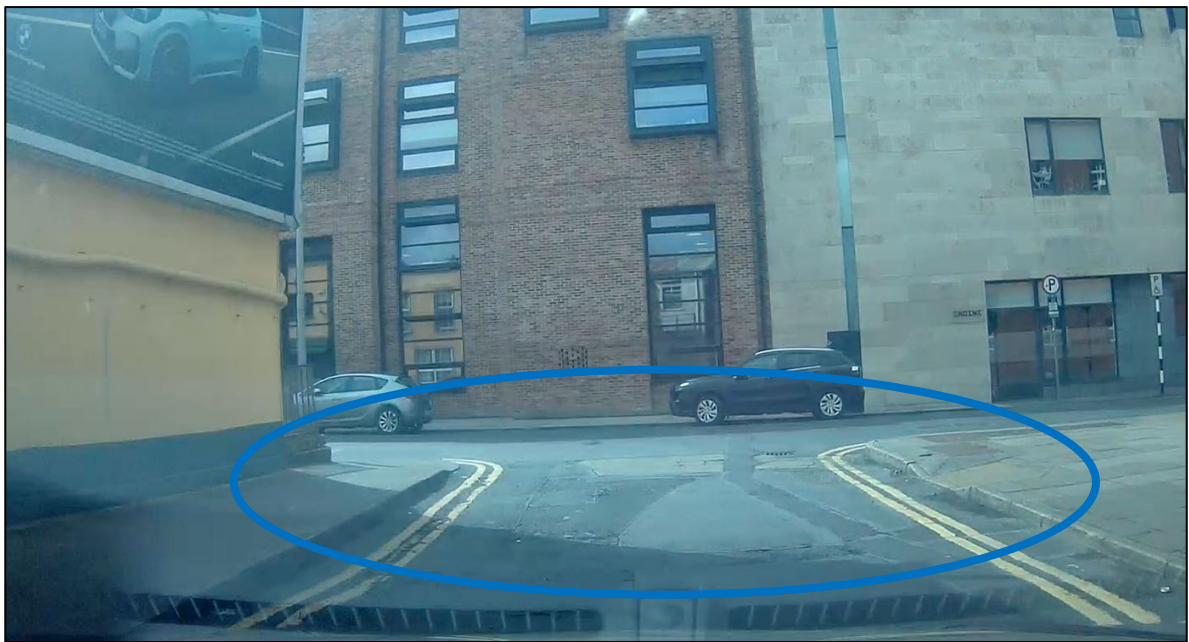
Figure 2.4 – Upstand Kerbs at Pedestrian Crossing
