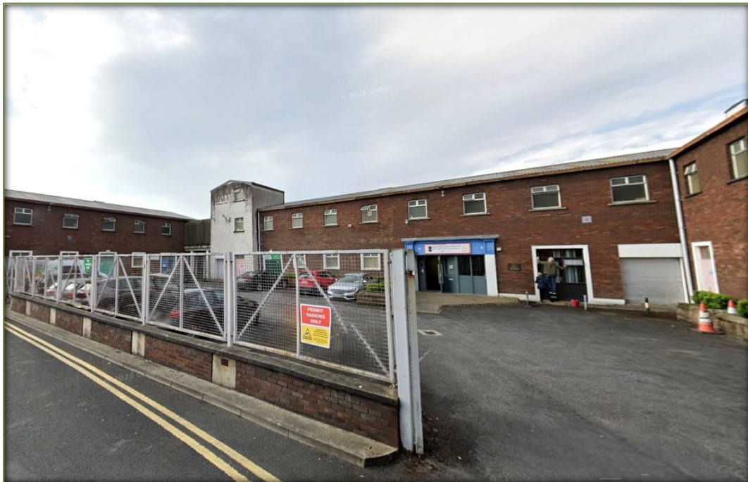
Figure 4b – Street View of the Site from Lady's Lane © Google
