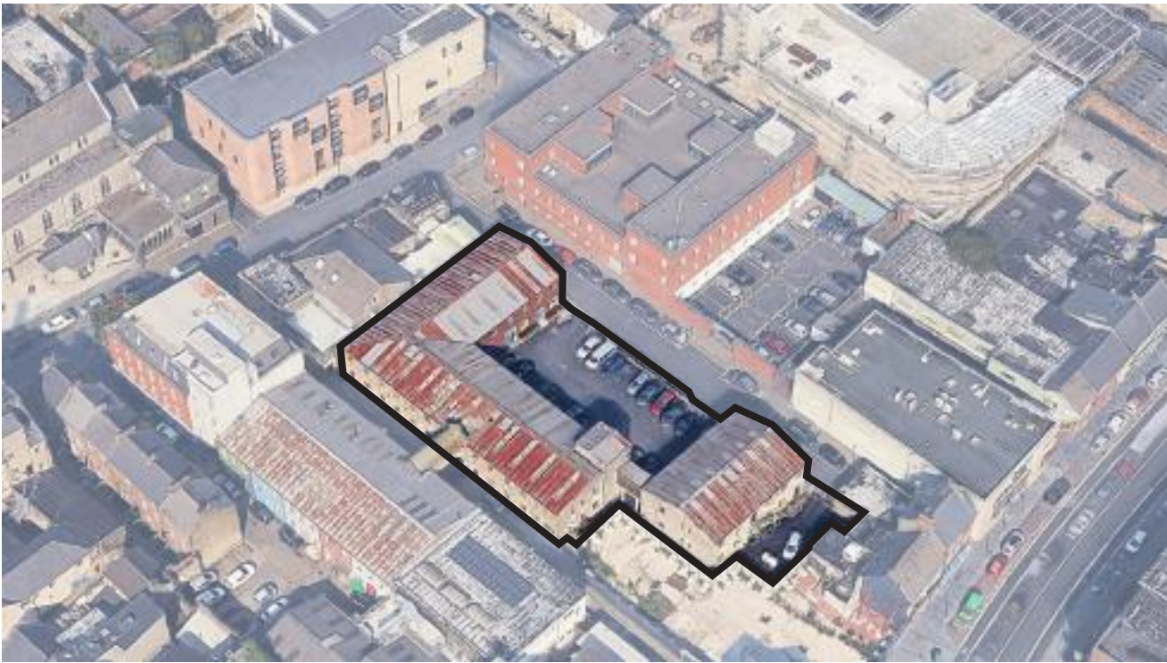
Aerial View looking Northwest
