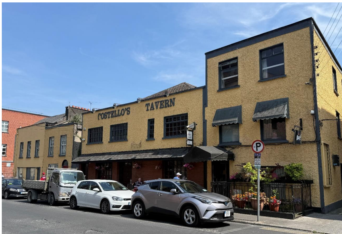
Fig. 7 Buildings fronting Baker Place
