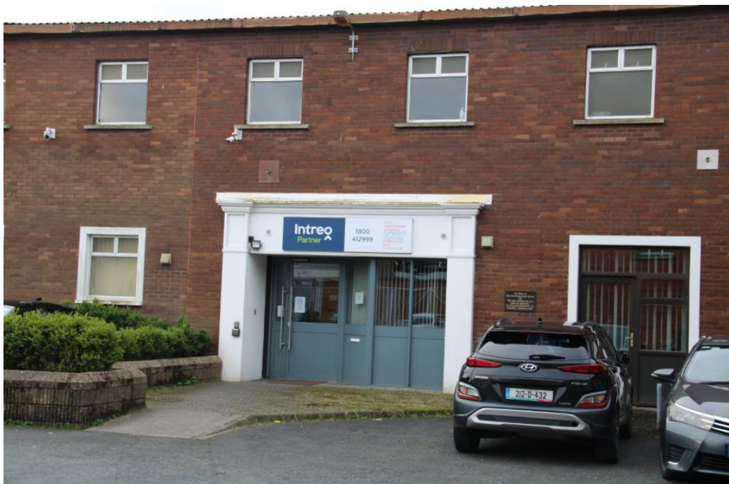
Fig. 6: Modern two-storey building on south side with red brick front façade. The roof appears to be corrugated iron. The building has two units with separate entrances.
