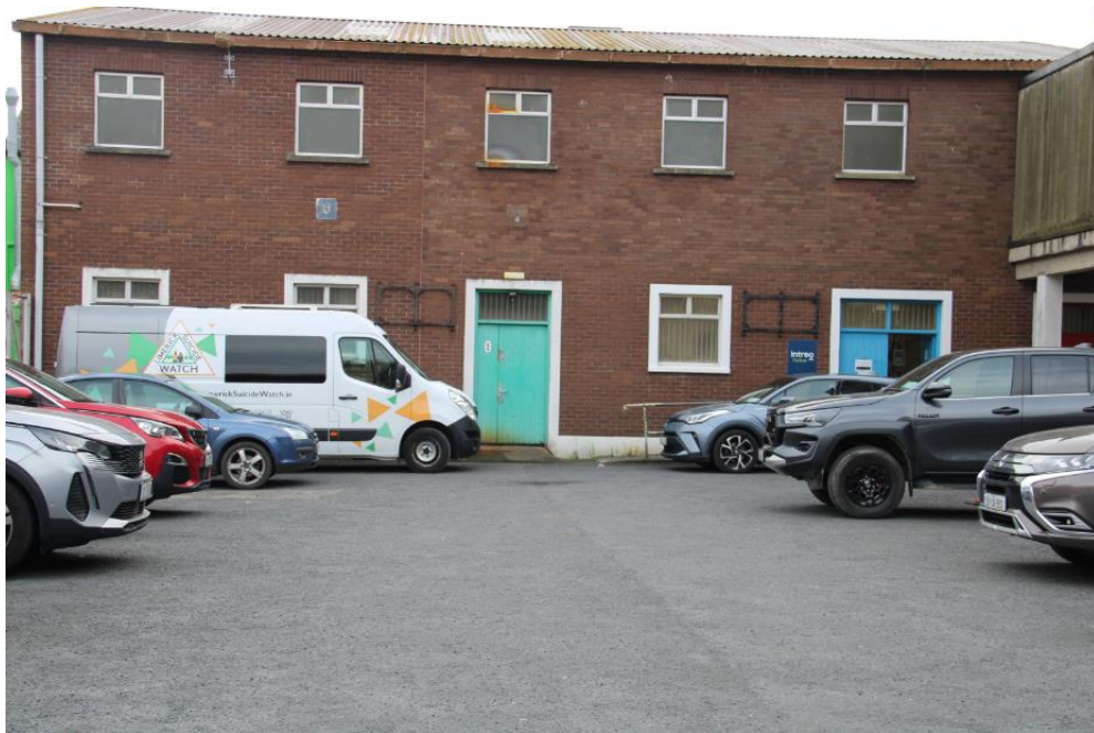
Fig. 4: Modern two-storey building on east side with red brick front façade and pebble-dash finish on the rear (west) side. The roof appears to be corrugated iron. The building is in two units with separate entrances.
