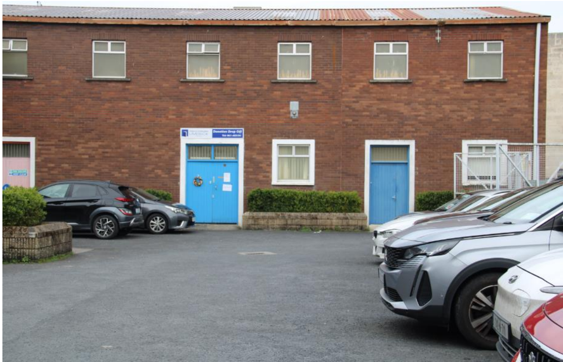
Fig. 5: Modern two-storey building on west side with red brick front façade. The roof appears to be corrugated iron. The building is in three units with separate entrances.
