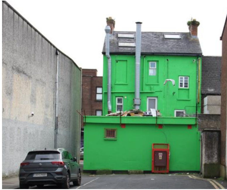
Fig. 9: Rear of building at junction of Lady's Lane and Parnell St.
